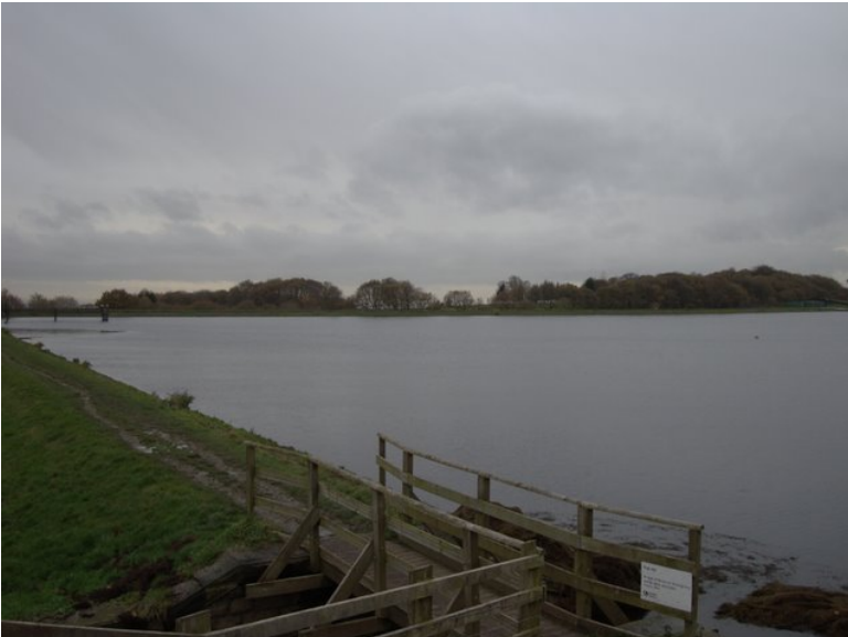
More of the same, viewed from the pump house. (Ian McKerchar)
