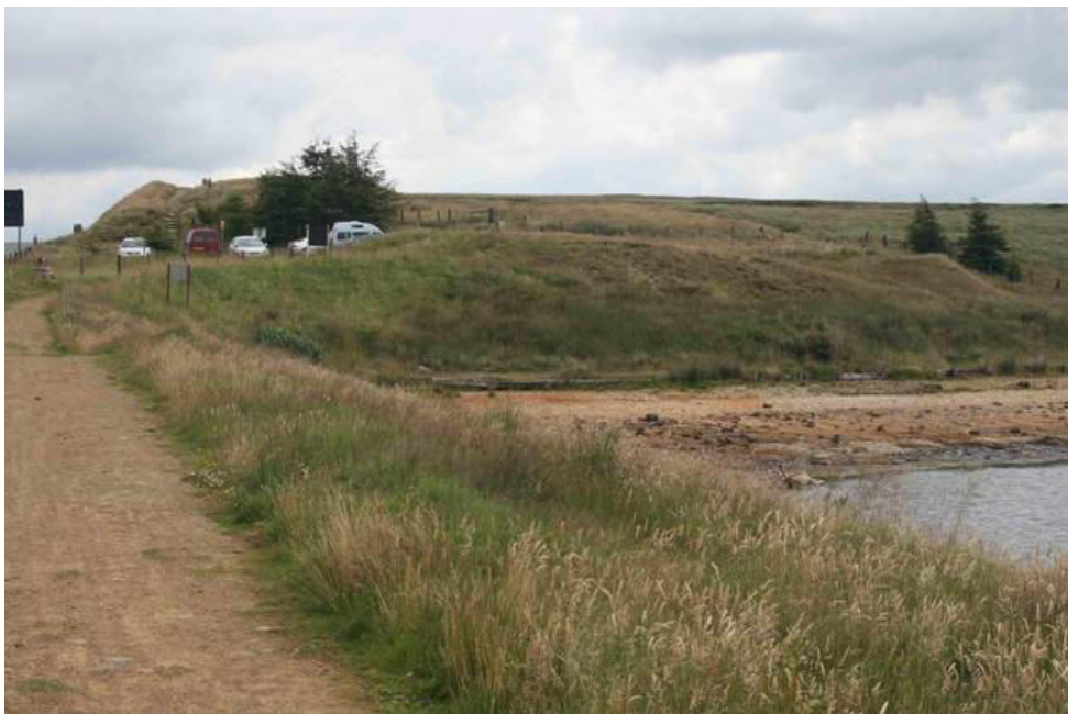
View looking east towards the car park. In the distance, the Pennine Way and the back of the County boundary sign can be seen. (Photo by Mark Rigby)
